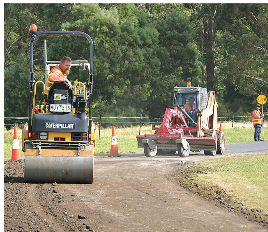
Above: After Polycom application, patch is levelled and rolled.
